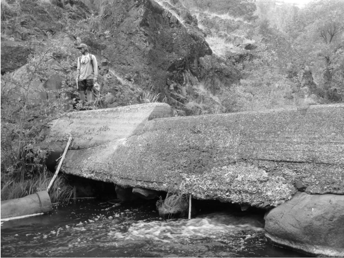
Figure 24 Dam structure in Jenny Creek, 1700 stream m from the confluence with the Klamath River, will potentially restrict fish movements upstream.
