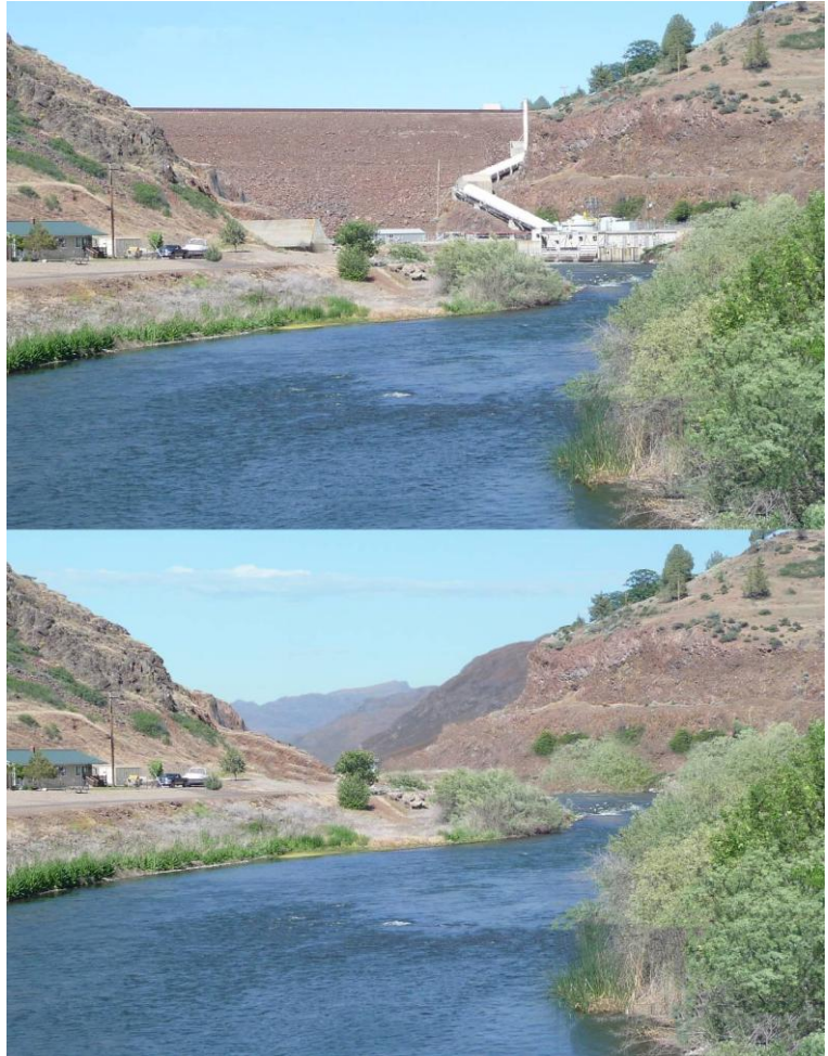
Figure ES-8. Simulation of Iron Gate Dam Before and After Full Facilities Removal
