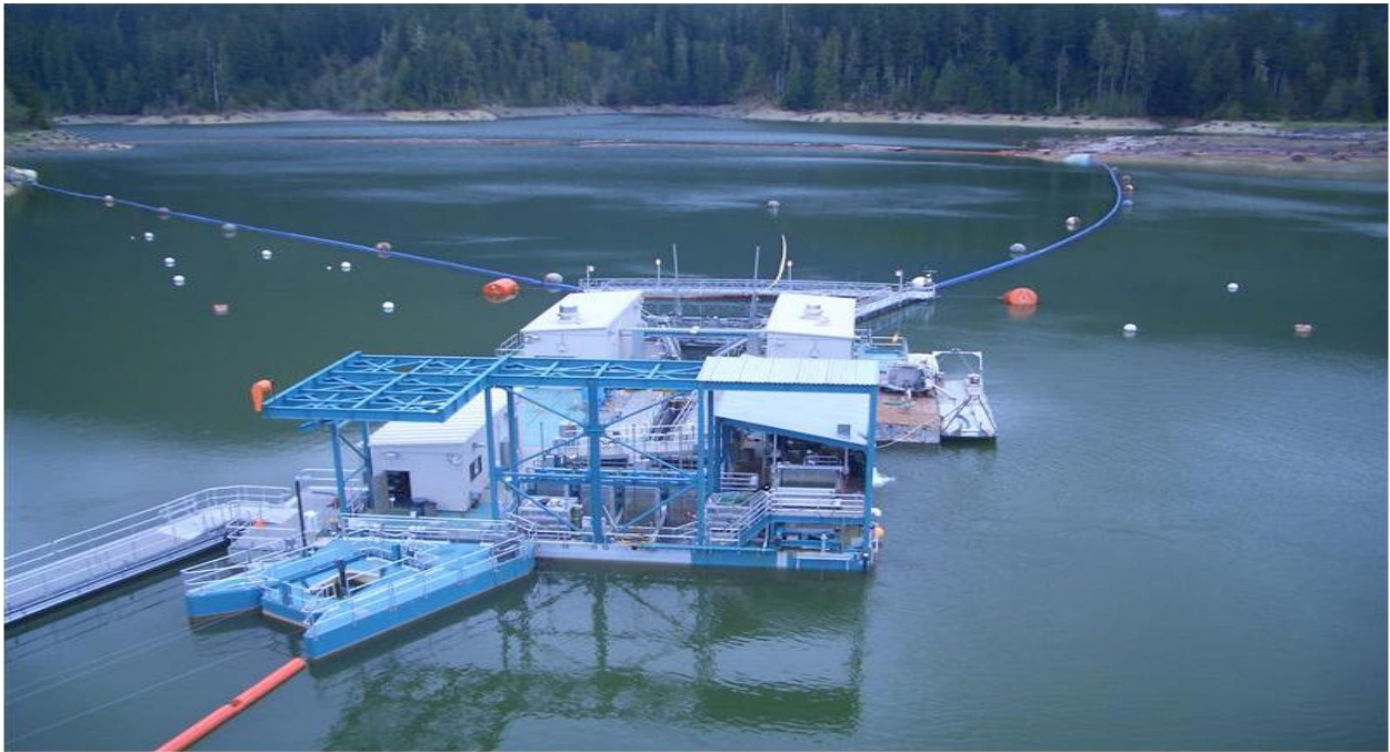
Figure 2-25. Example of Floating Surface Bypass Collector in Upper Baker Dam, Washington
