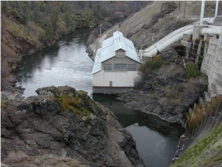
Figure 1-4: Copco 1 Dam, powerhouse, and downstream area of the Klamath River. This facility would be removed under the KHSA.
