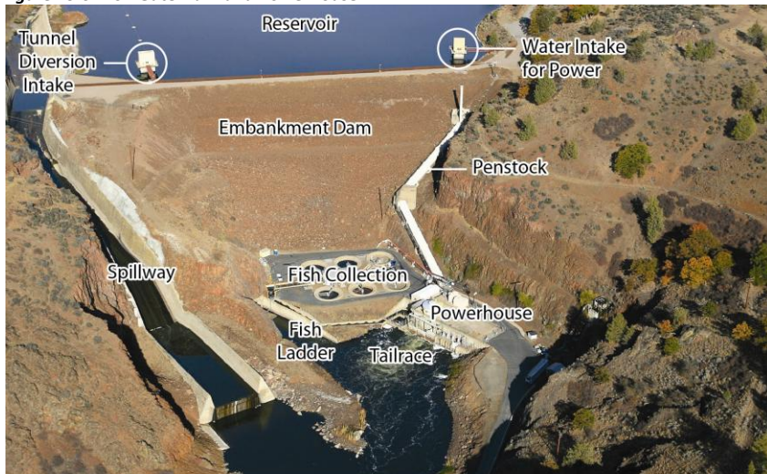
Figure ES-6: Iron Gate Dam and Powerhouse
