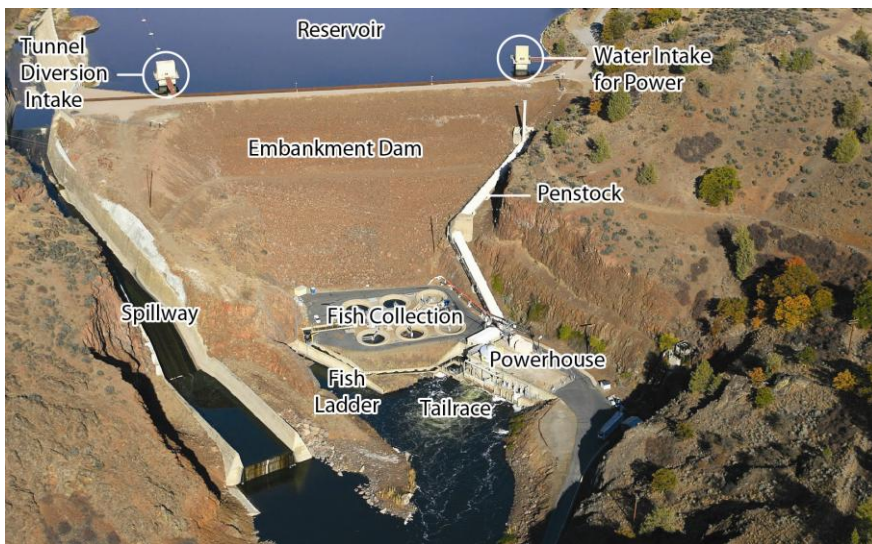
Figure 4.2-10: Photo of Iron Gate Dam and Reservoir with Specific Components Labeled. With full facilities removal, all visible components would be removed. With partial facilities removal, certain components (e.g., penstock) would be retained.
