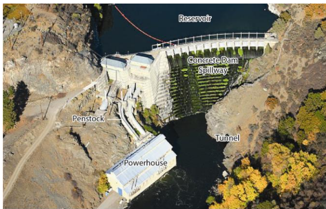
Figure 4.2-5: Photo of Copco 1 Dam and Reservoir with specific components labeled. With full facilities removal, all visible components would be removed. With partial facilities removal, certain components (e.g., penstock) would be retained.
