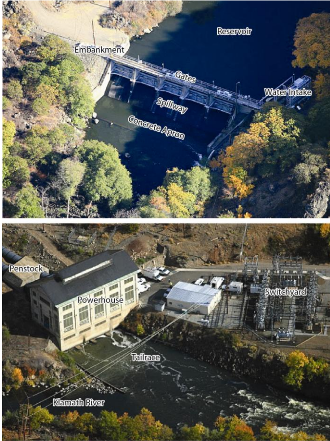
Figure ES-5: Copco 2 Dam and Downstream Powerhouse
