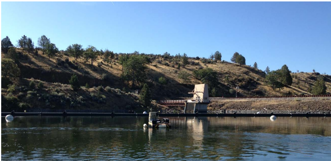
Figure 31. Autosampler Located Upstream of the Curtain in Iron Gate Reservoir.
