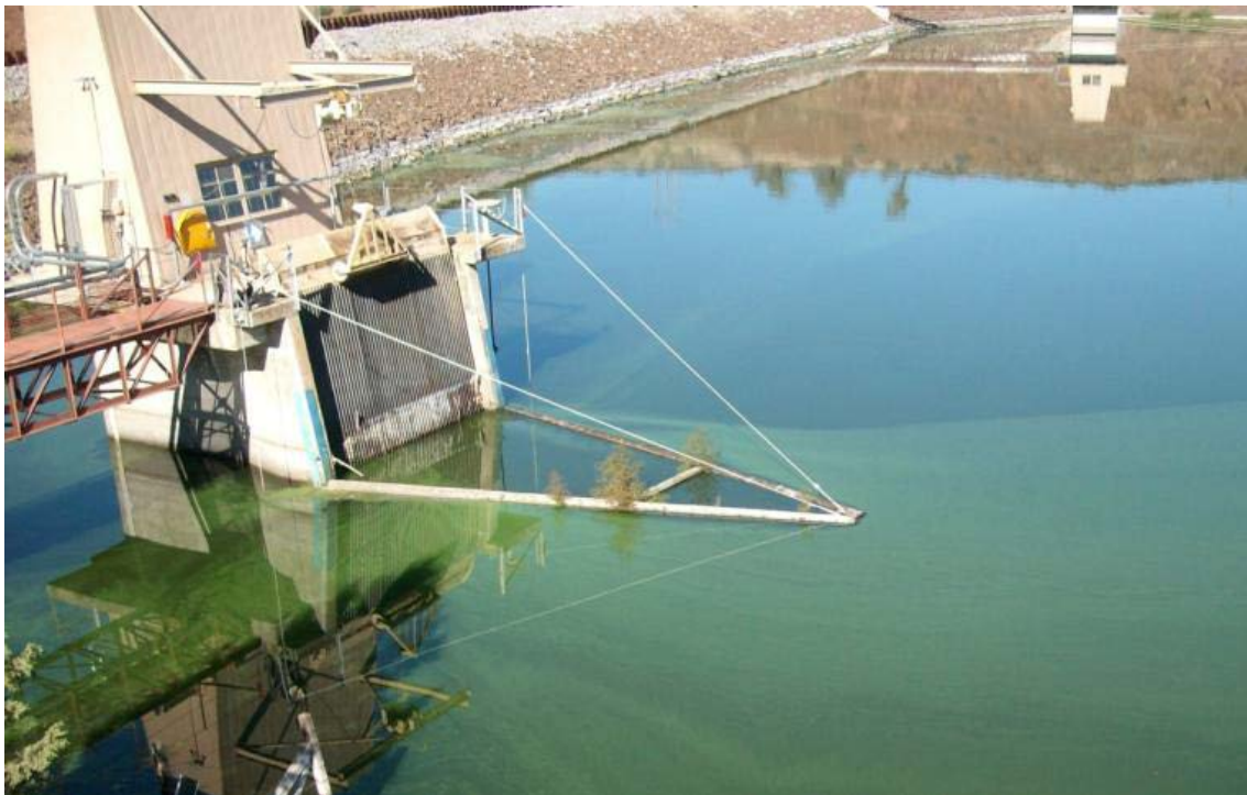
Figure 1. Iron Gate Reservoir Intake Tower, Trash Rack, and A-frame Debris Boom.
